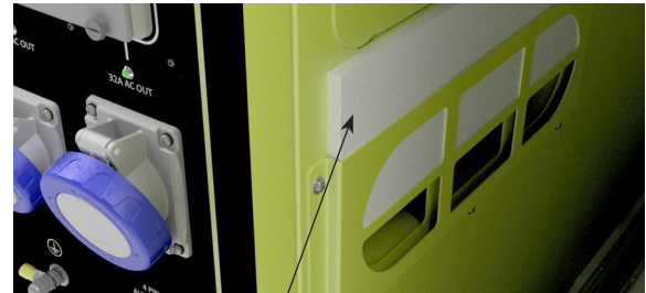
Slide up foam mesh to change filter
